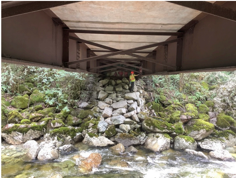
Left Bank Abutment when facing downstream
