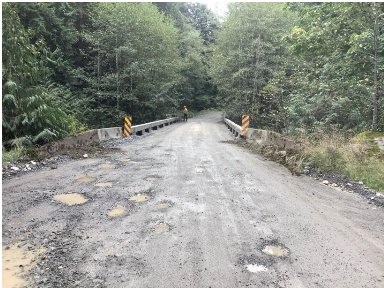
Approach from Right Bank when facing downstream
