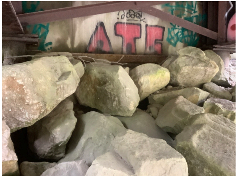
Left Bank Abutment when facing downstream
