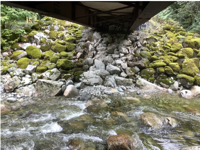
Right Bank Abutment when facing downstream
